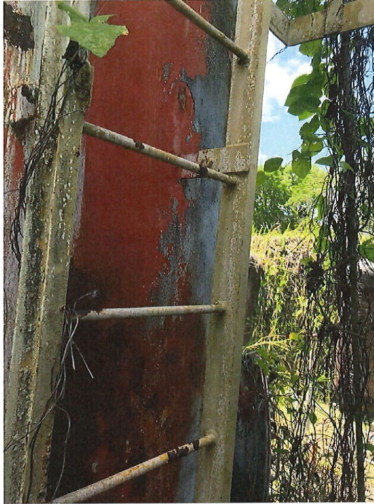
Photo Number 32 – Building Exterior Tank Stairs
