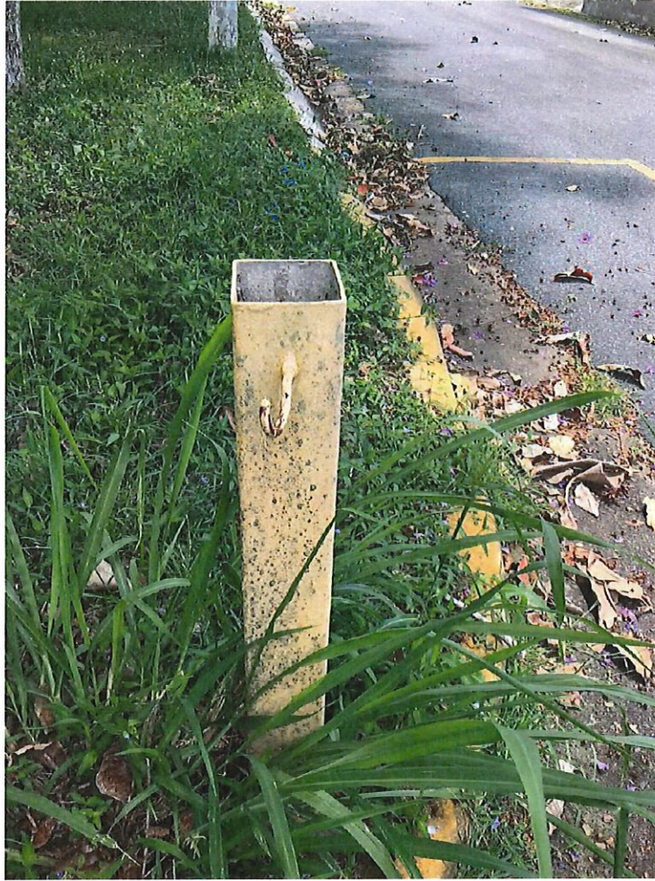
Photo Number 37 – Building Exterior Parking Bollard
