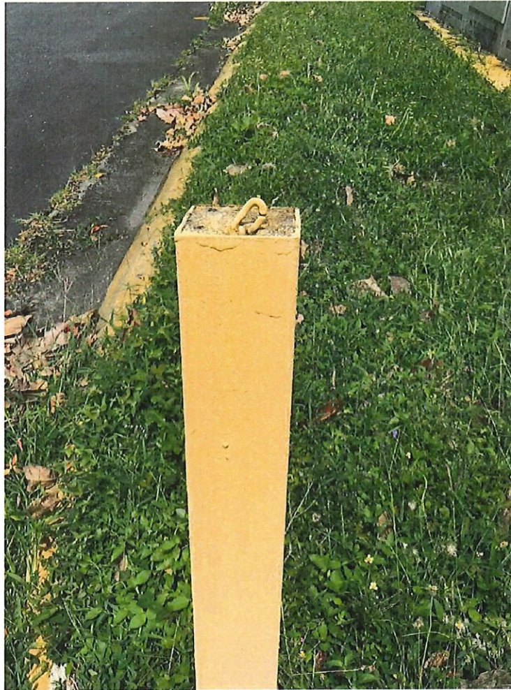
Photo Number 36 – Building Exterior Parking Bollard
