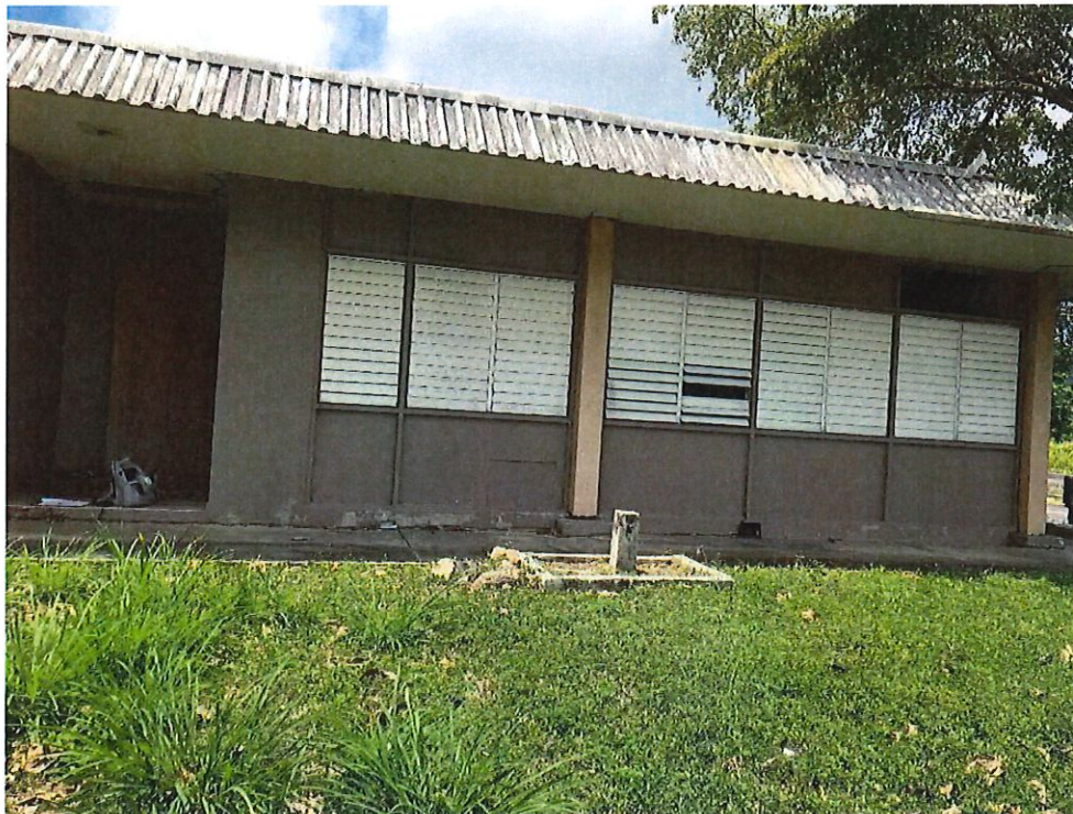
Photo Number 2 – Exterior Walls
