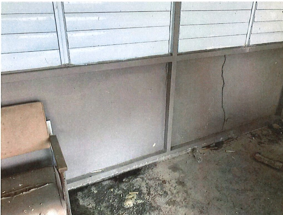
Photo Number 31 – Wall Interior "A" Loading Platform
