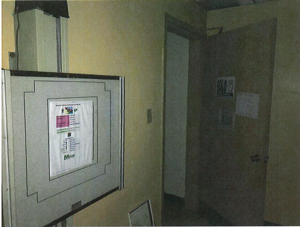
Photo Number 27 – Wall “C” Interior X-Ray Room
