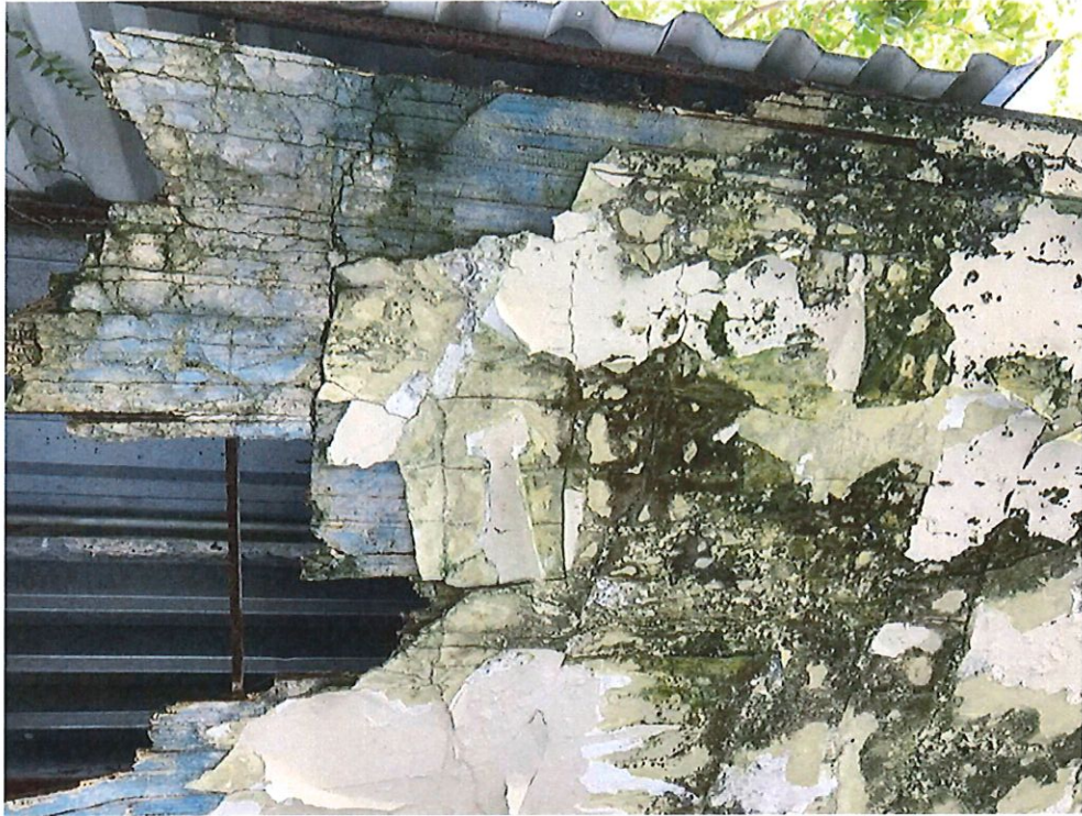
Photo Number 1 – Alero Building exterior, Wall “B”
