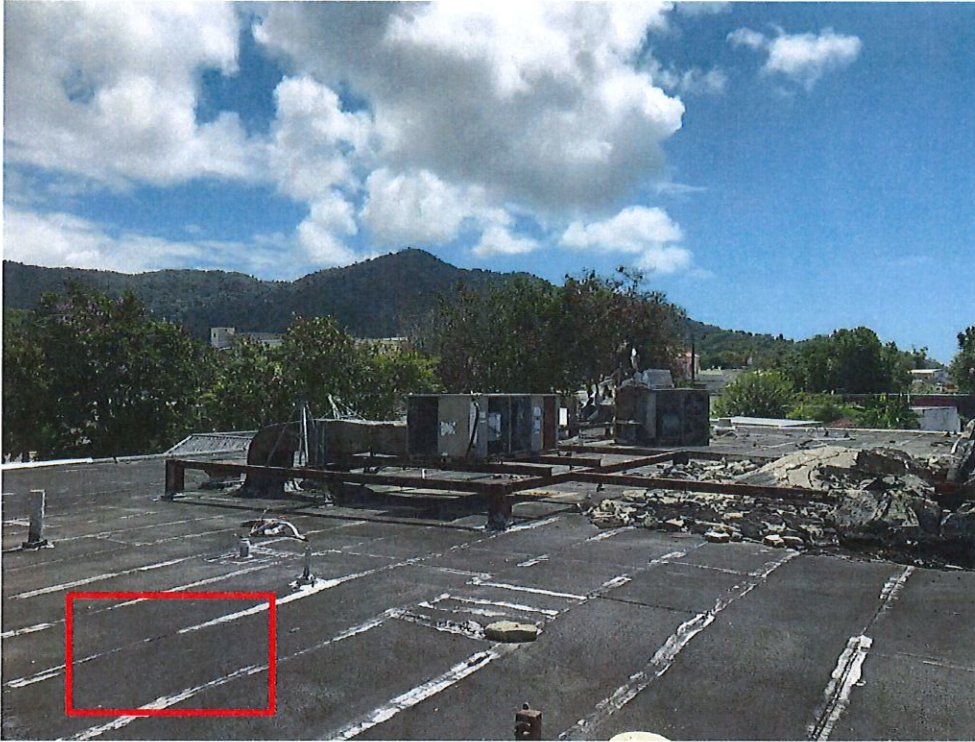
Photo Number 10 – Roof Treatment
