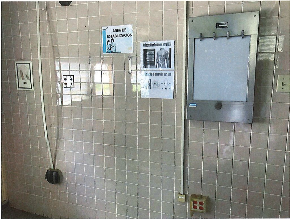
Photo Number 22 – Wall Interior Emergency Room
