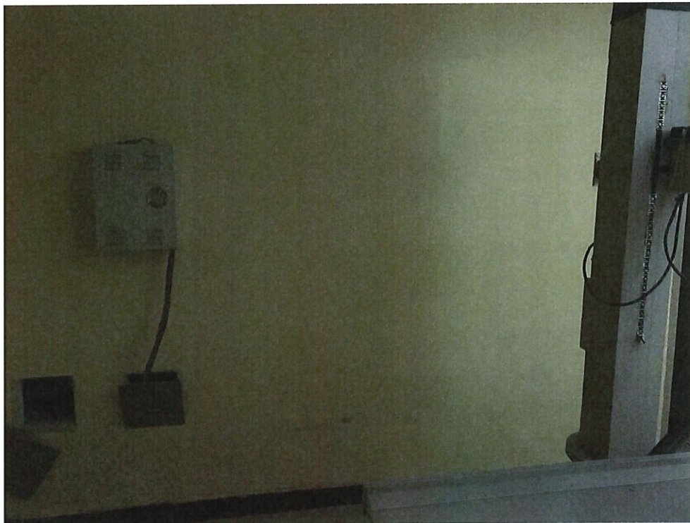
Photo Number 26 – Wall “D” Interior X-Ray Room
