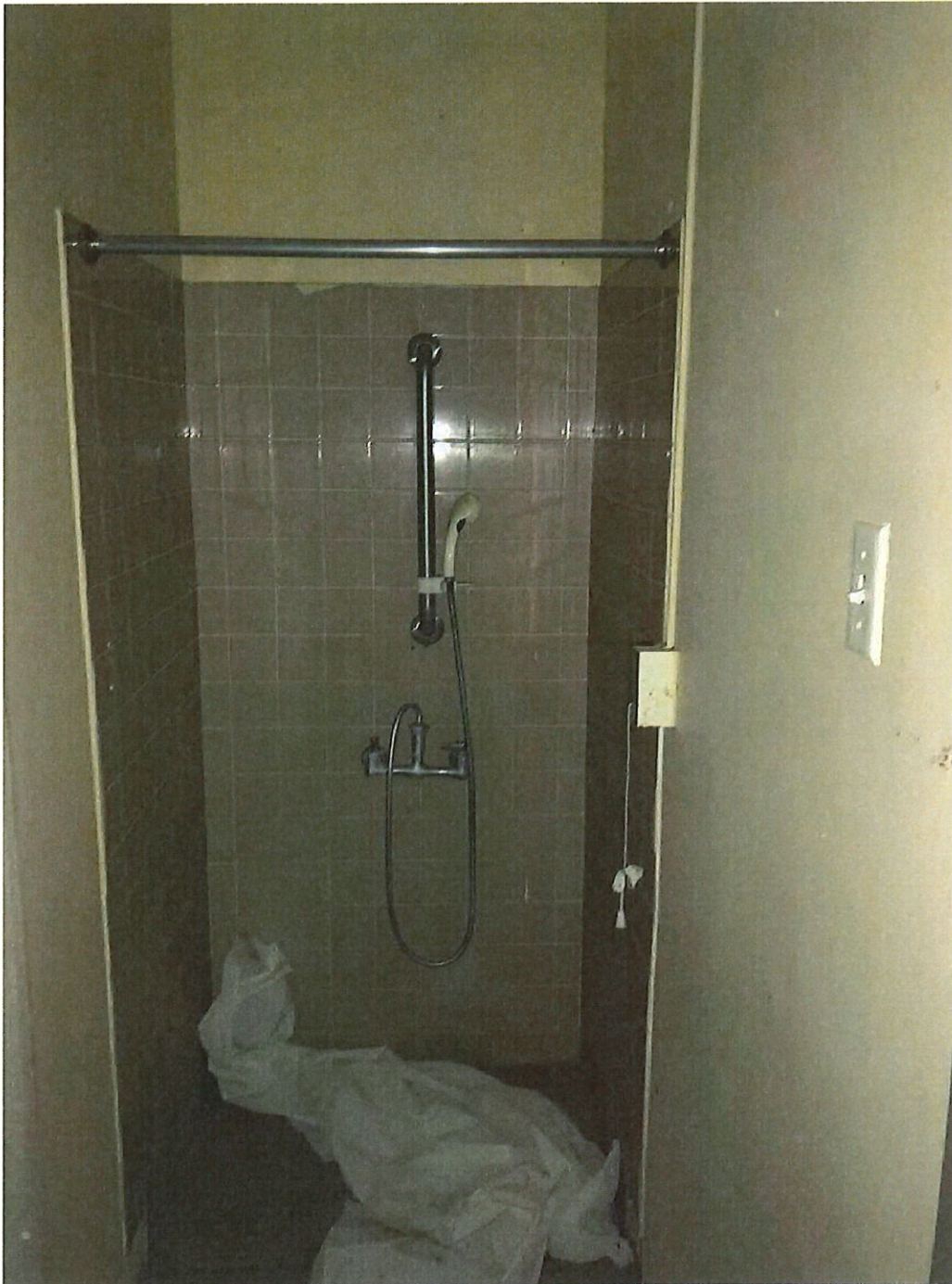
Photo Number 20 – Wall Interior Jan (Janitor) Room 58D
