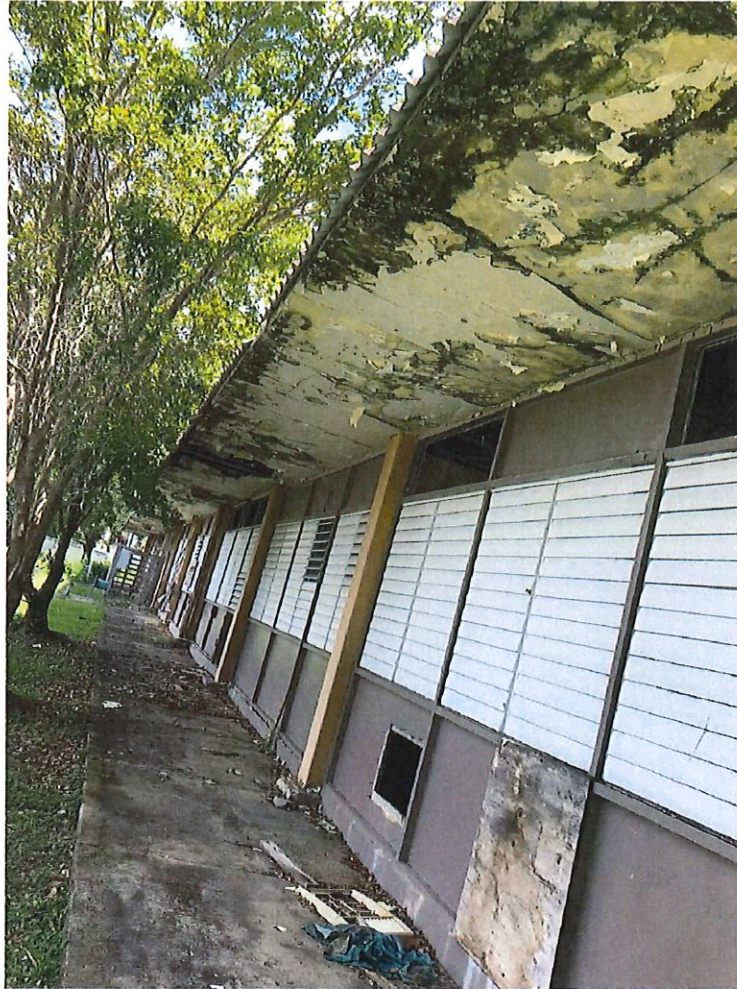
Photo Number 2 – Alero Building Exterior, Wall “C”
