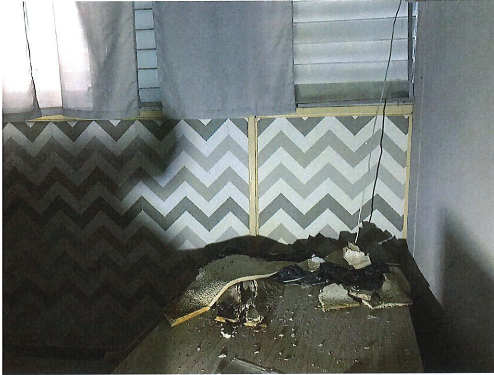
Photo Number 16 – Wall Interior “A” Exam & Treatment Room (83C)
