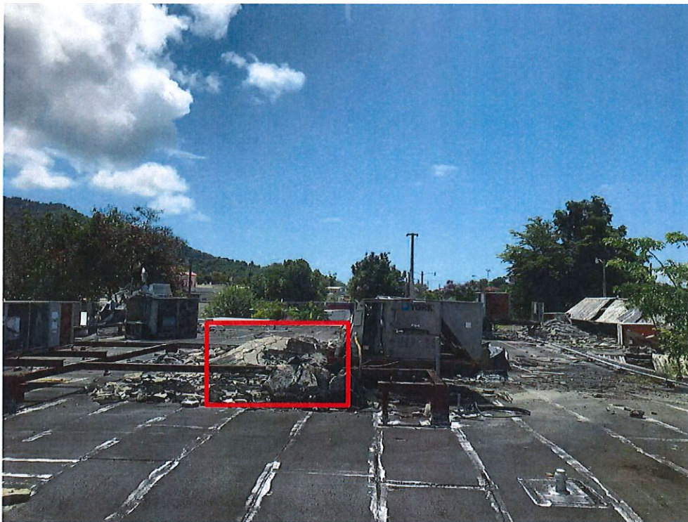
Photo Number 11- Roof Concrete
