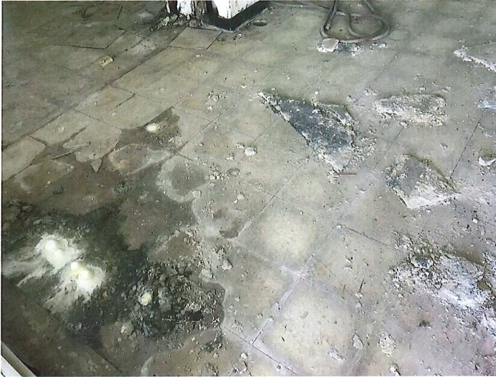
Photo Number 5 – Work Area Floor Tiles
