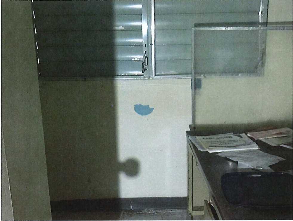
Photo Number 21 – Wall Interior “A” Soiled Utility
