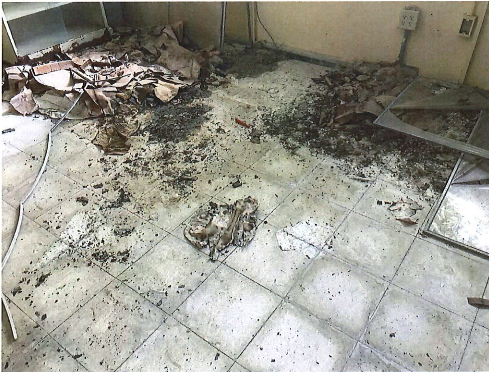
Photo Number 6 – Information Room Floor Tiles
