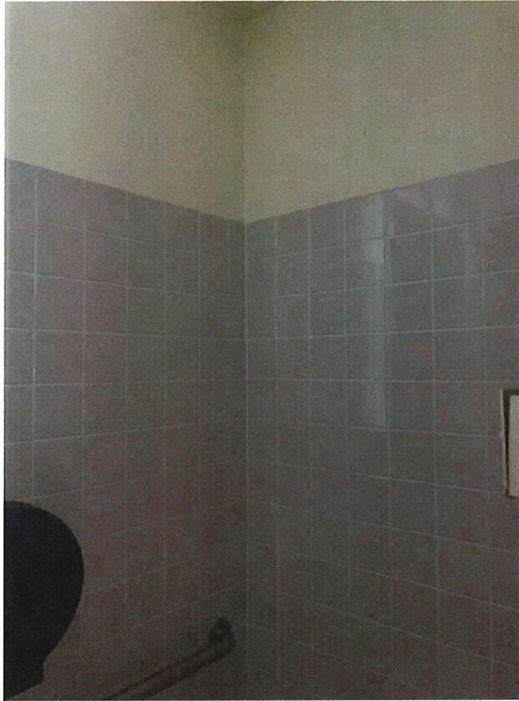
Photo Number 15 – Wall Interior Restrooms
