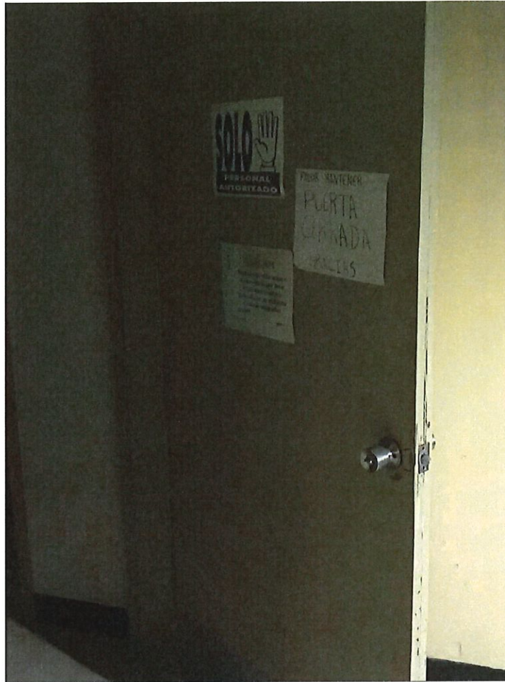
Photo Number 28 – Door Frame and Door Interior X-Ray Room
