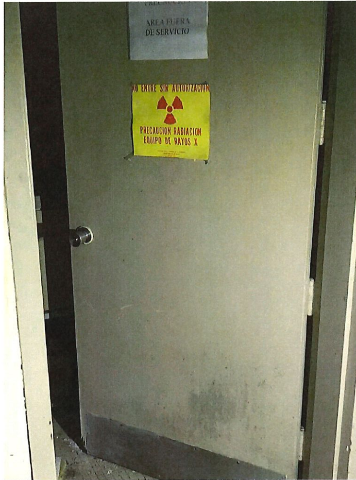
Photo Number 24 – Door Frame and Door Interior X-Ray Room
