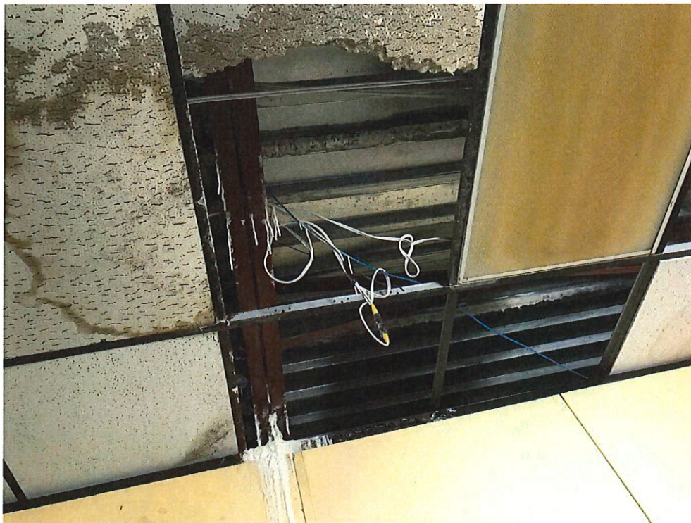
Photo Number 8 – Exam & Treatment Room Acoustic Ceiling
