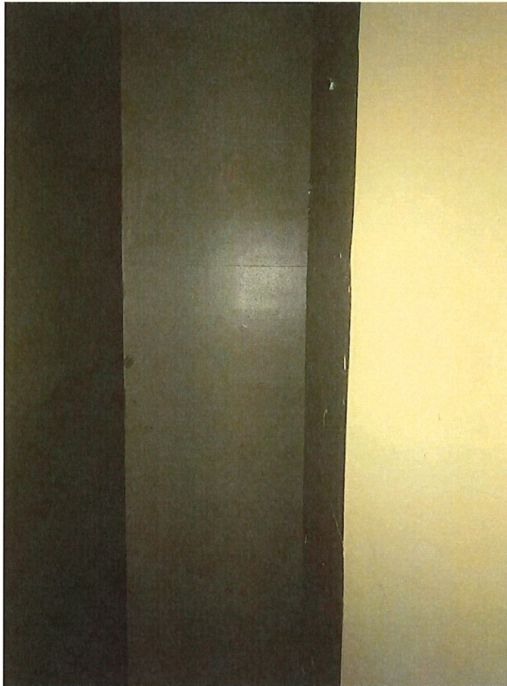
Photo Number 29 – Wall Interior Control X-Ray Room
