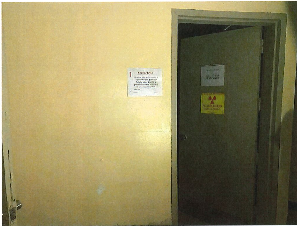
Photo Number 23 – Wall Interior “A” X-Ray Room
