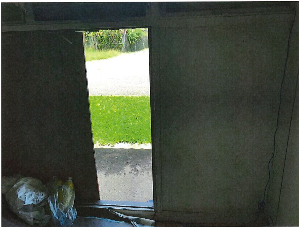
Photo Number 17 – Wall Interior “A” Exam & Treatment Room (71C)
