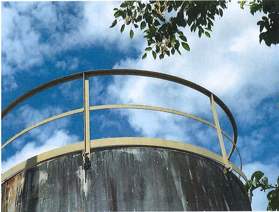
Photo Number 33 – Building Exterior Tank Handrail
