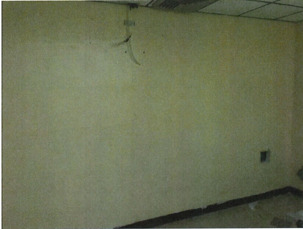
Photo Number 25 – Wall “B” Interior X-Ray Room
