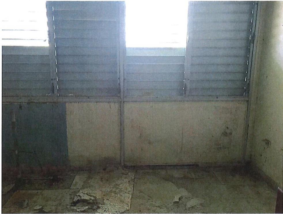
Photo Number 13 – Wall interior “D” Work Area
