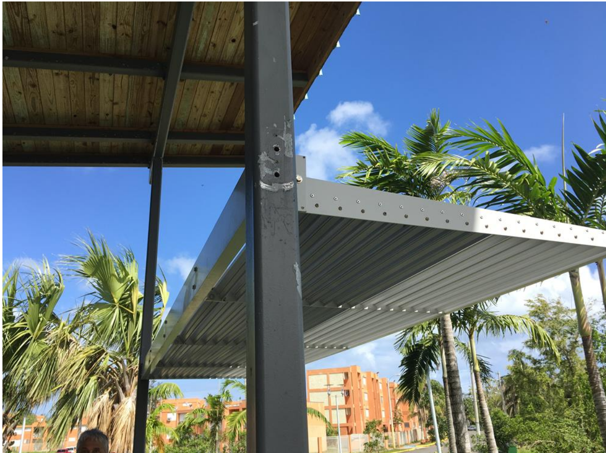
Photo 5. Exhibition Center's trellis broken
