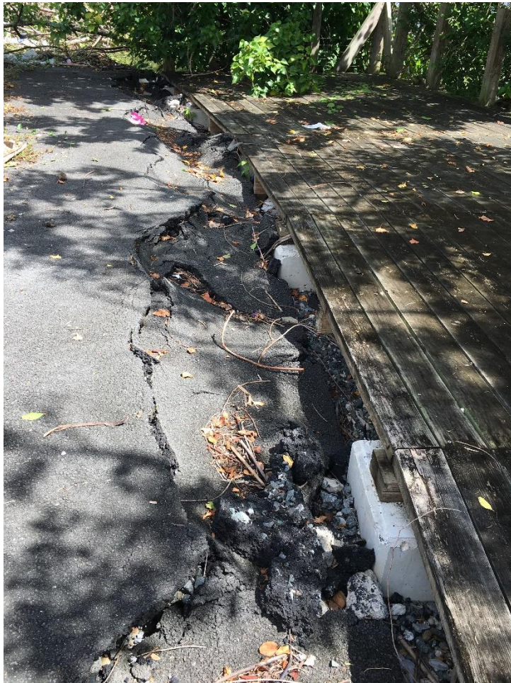
Photo 6. Water and flood undermined pavement
