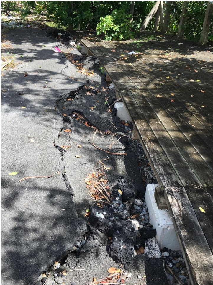
Photo 6. Water and flood undermined pavement
