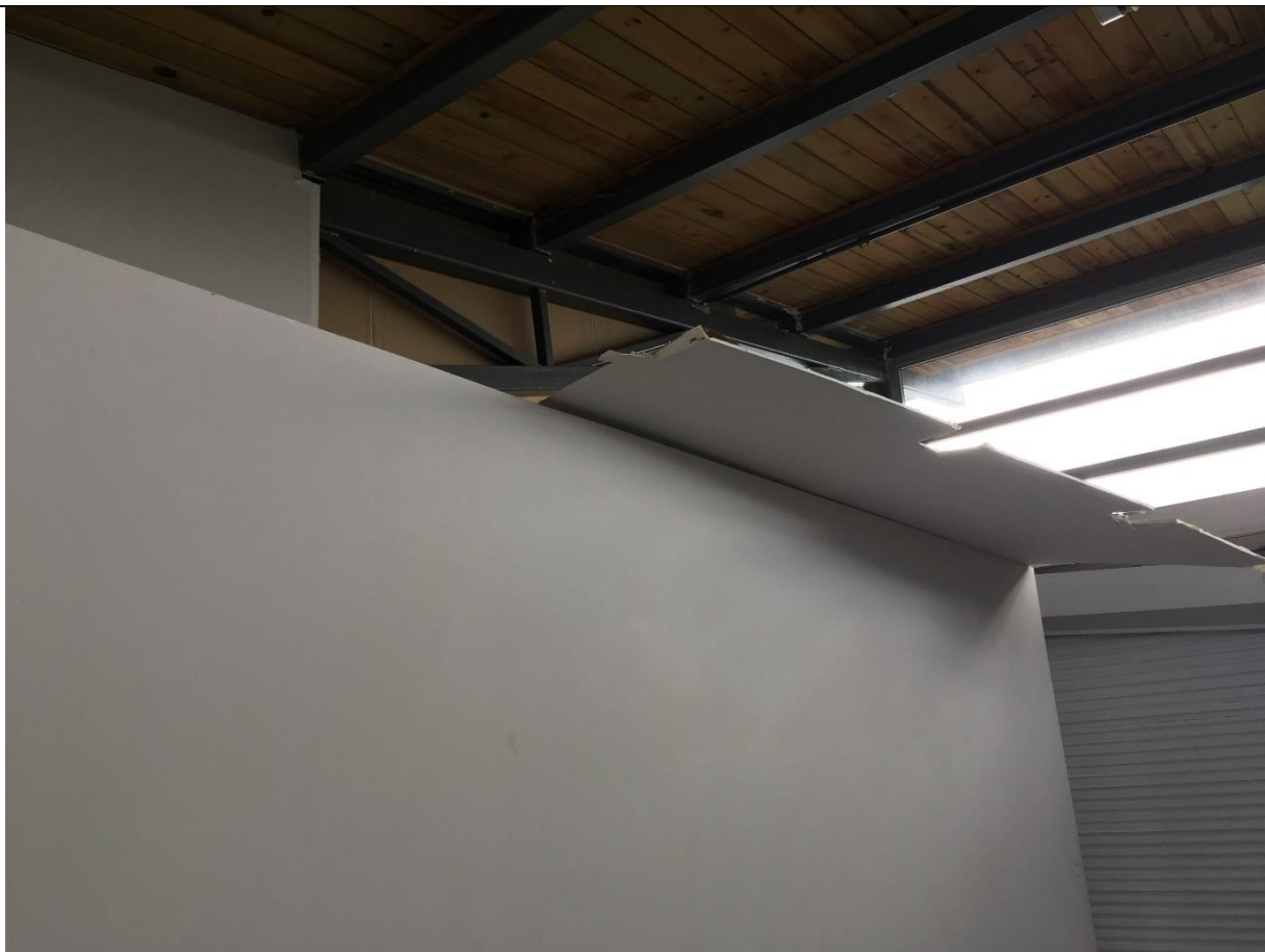
Photo 4. Audiovisual Center gypsum board wall damaged
