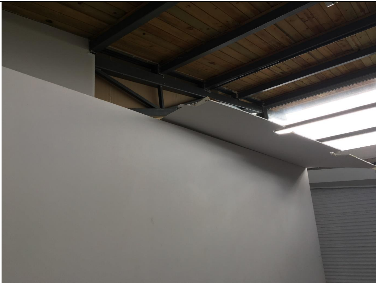
4. Audiovisual Center gypsum board wall damaged
