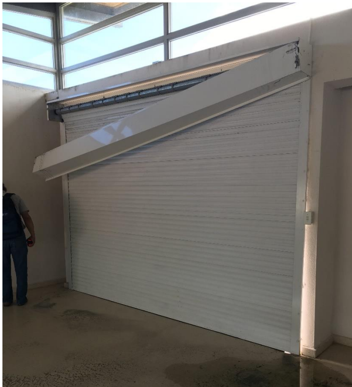
Photo 3. Restaurant's rolling doors damaged
