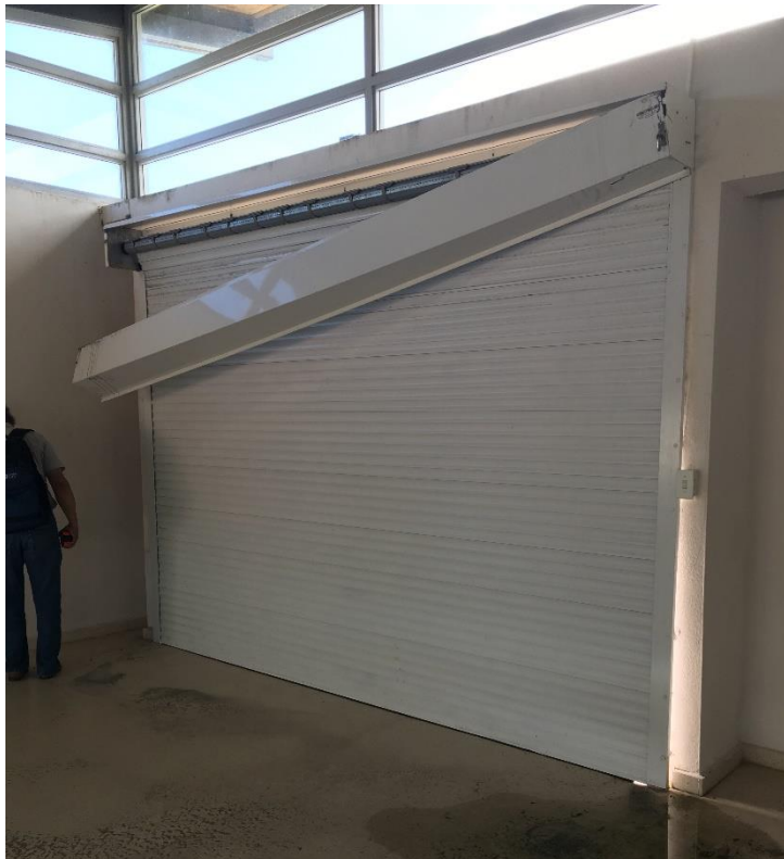
Photo 3. Restaurant's rolling doors damaged
