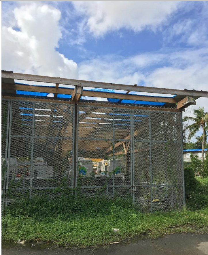
Photo 2. Utility building's roof damages
