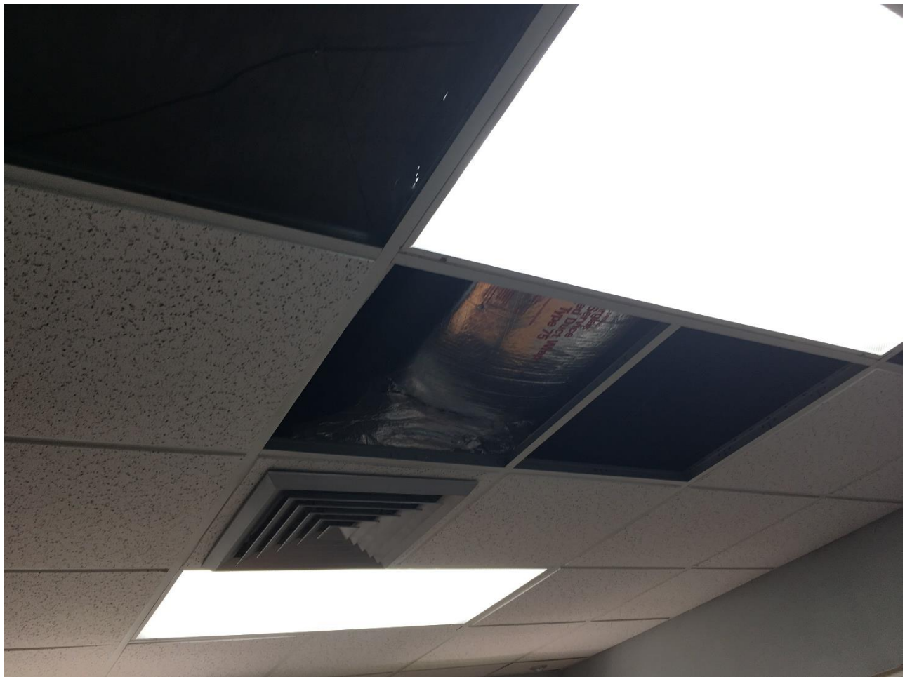
Photo 1. Community Center A/C and Acoustical Ceiling Damages
