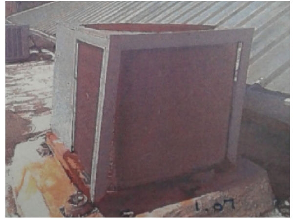
Site2: A/C condensing units 7.5 Ton
