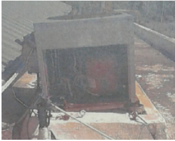
Site 2: A/C condensing units 1.5 Ton
