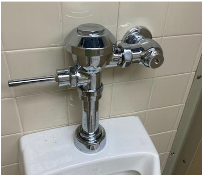
Typical Chrome Metal Urinal Valve Painted with LBP Men Bathroom
