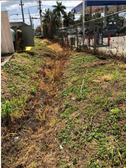
Photo #9: Stormwater Earth Swale
