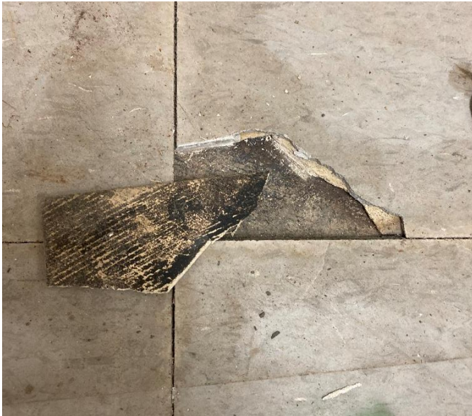
Typical Asbestos Containing VFT/Mastic
