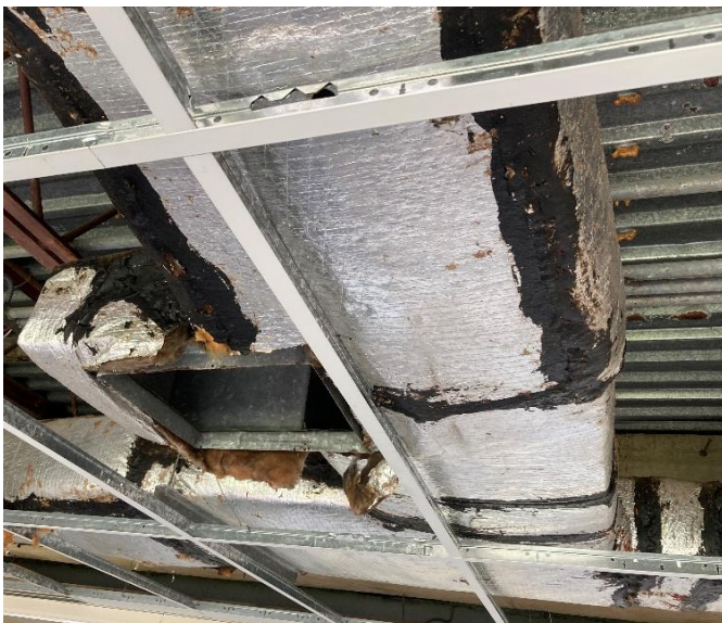
Typical Asbestos Containing Mastic on HVAC Ducts present in Classroom and Administration Area
