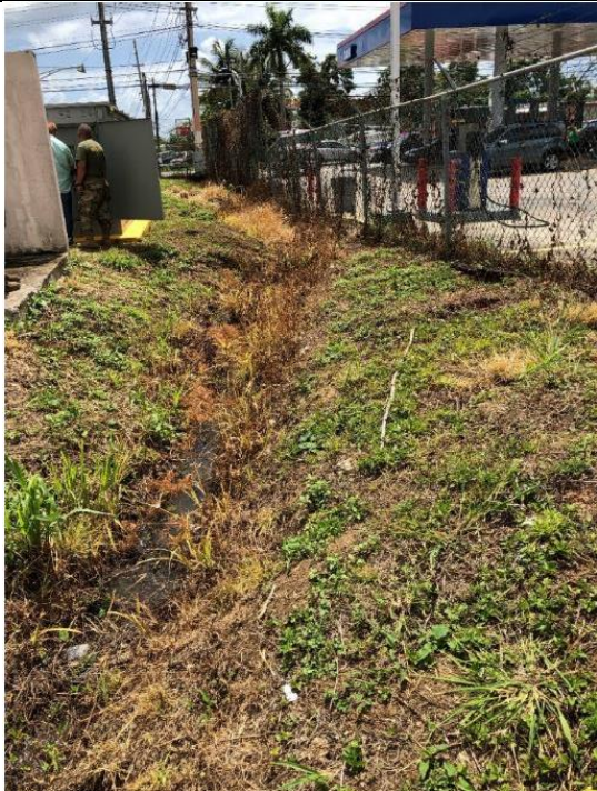
Photo #9: Stormwater Earth Swale
