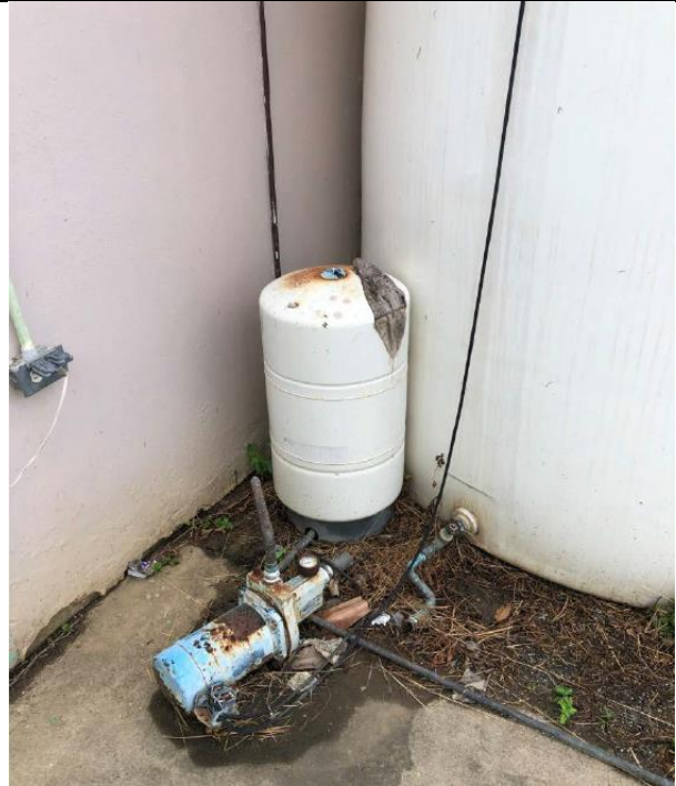
Photo #14: Water Cistern & Hydro-Pneumatic Tank
